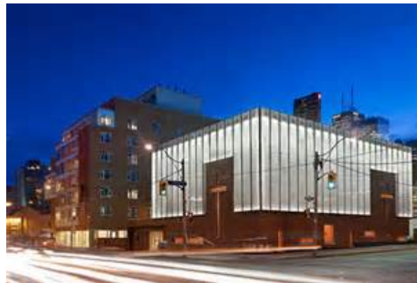
Harbour Light Ministries, 160 Jarvis Street, Toronto
